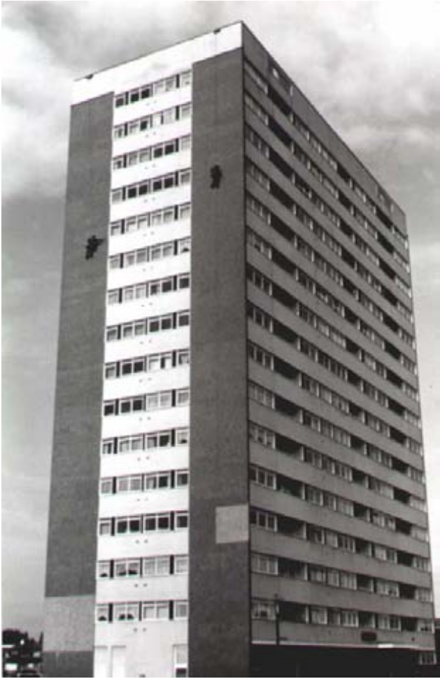
Flats being checked by 'spidermen' workers.....
