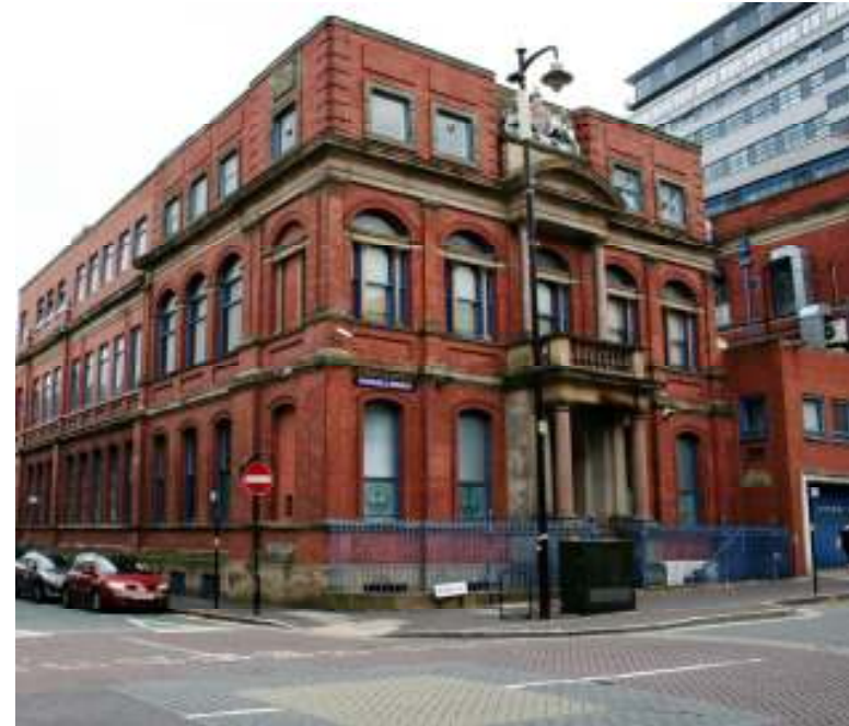
Above: Birmingham Assay Office in its current home on Newhall Street where it has been for 135 years. A new building is underway and the assay office will be moving in 2014
