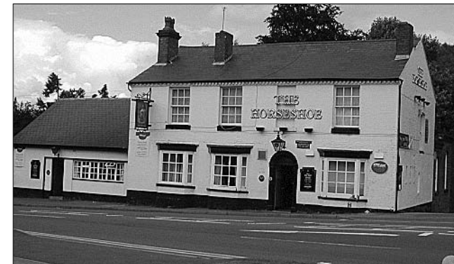
The Horseshoe PH - Alcester Road South
