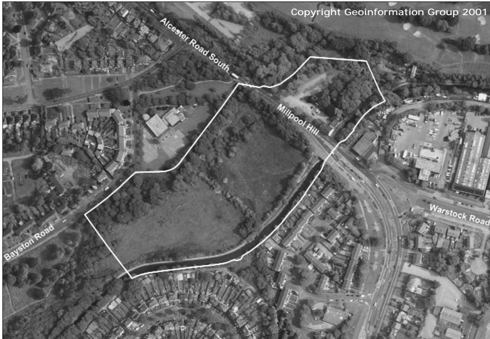
Aerial view of of the Development Brief area
