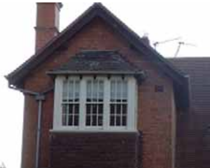
Bournville: Elevation detail
