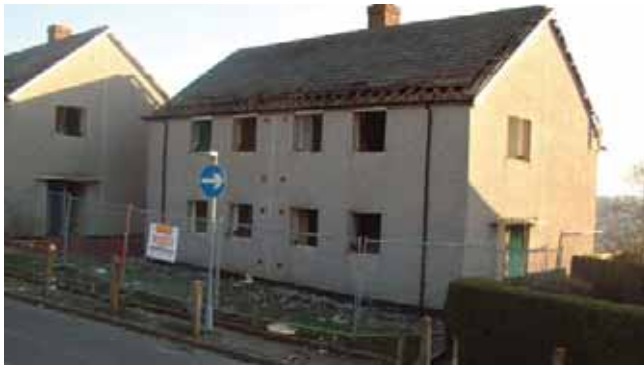
Demolition and redevelopment
