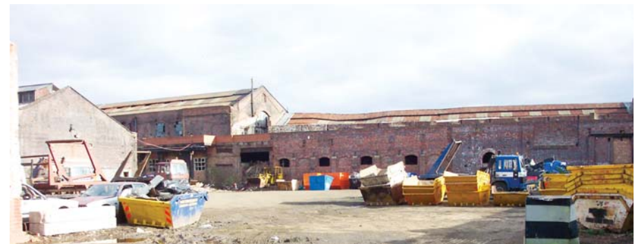
Derelict site at Icknield Port Loop
