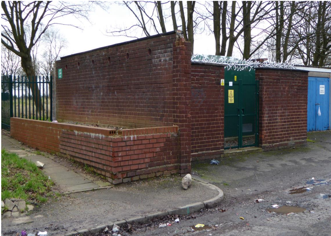
Plot 18 – existing substation 5067 to the east of the Poolway.
