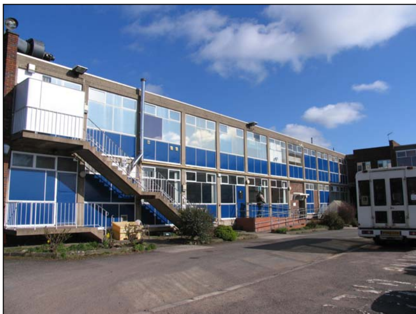
A day centre building
