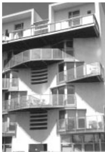
Features such as balconies can increase amenity space and add liveliness and interest.
