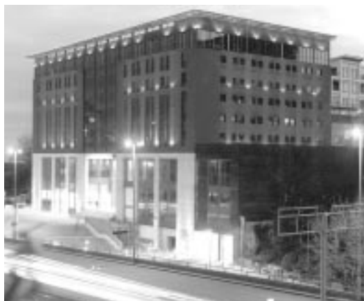
Many developments are a positive step forward. The Mailbox - housing as part of a mixed use development.
