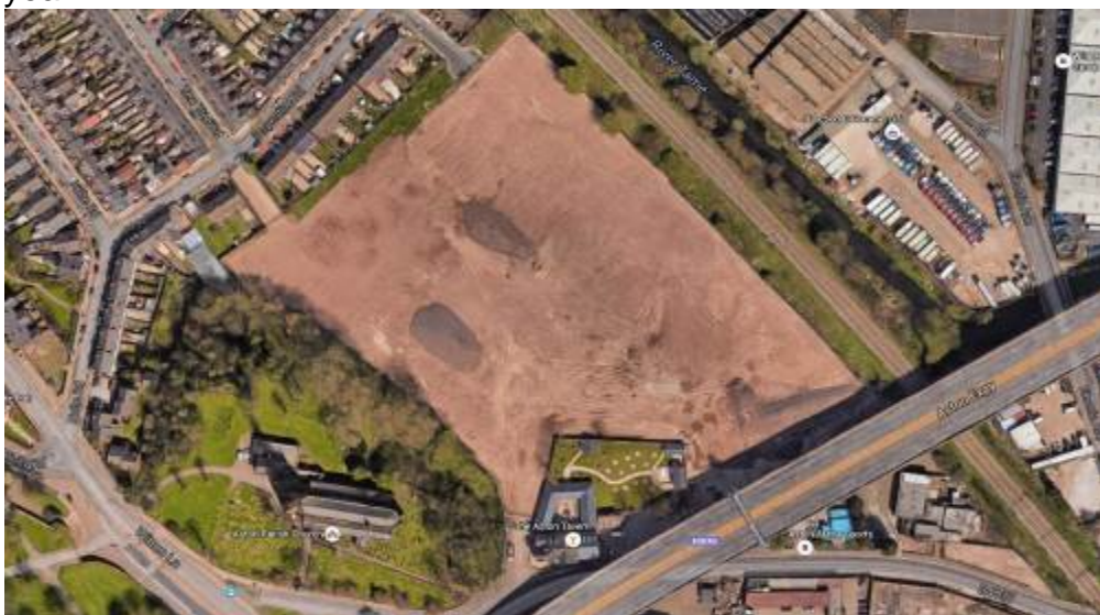
Figure 4: Ariel photo of Area 2 of the site.
