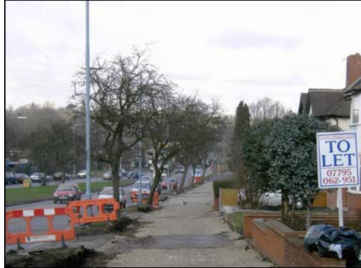
Existing Hawthorn trees just after the laying of the hardcore
