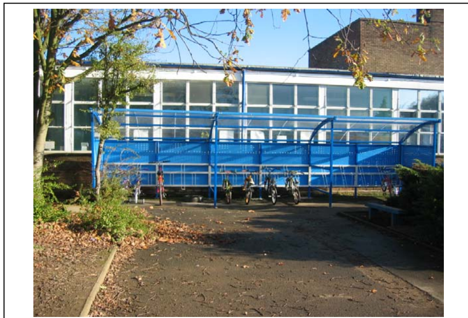
Making cycling a practical alternative: Modern, open cycle storage introduced at Four Dwellings Primary School, Quinton.
