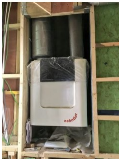
Image of Zehnder MVHR unit being retrofitted into an existing house (Source: Bow Tie Construction)
