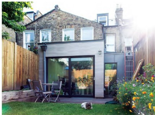
EnerPHit retrofit project with extension (Source: Passivhaus Plus)
