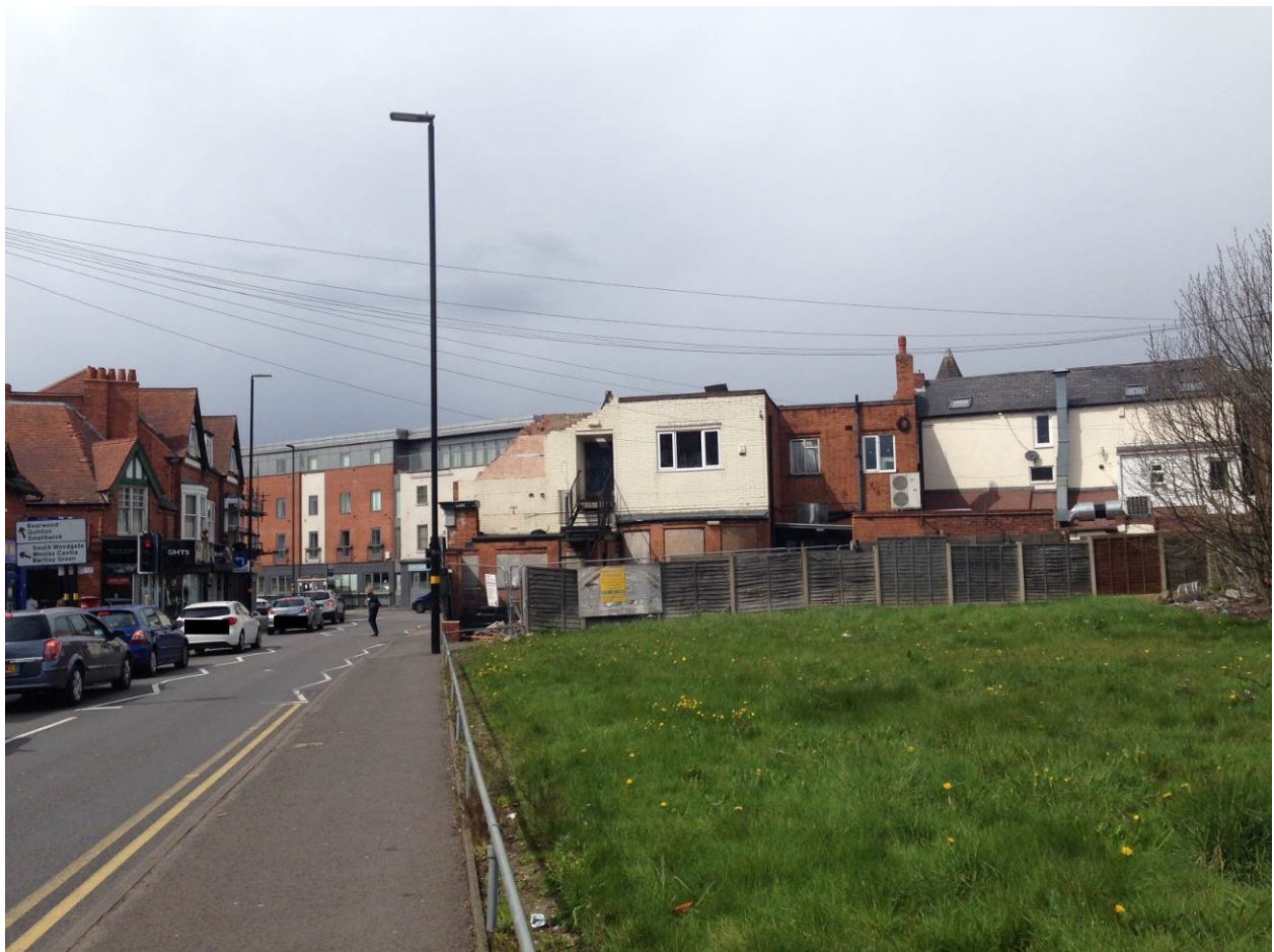
Photo 2: View from south on Harborne Park Road
