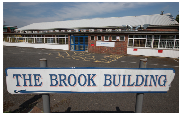
The site of the new Engineering Centre of Excellence in Redditch, North Worcestershire.
