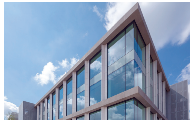
The new Joseph Priestly Building (BCU) at Eastside Locks. Image supplied by Goodman.
