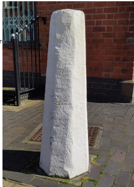
Image: Sandstone bollard (now painted), blue brick paviers, pink granite kerb, Vyse St Credit: Matthew Bott / JQDT
