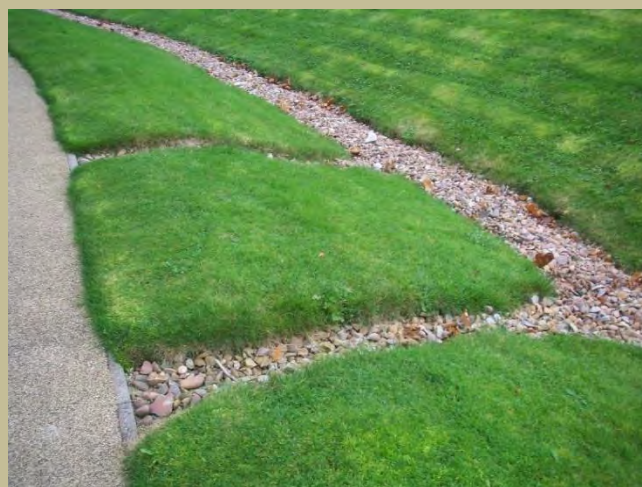
Example of a filter drain
