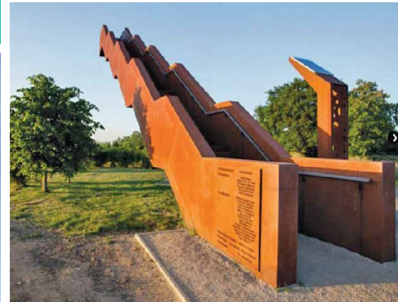
Example of cantilevered, sculptural staircase. Vlooyberg Tower, Tielt-Winge, Belgium. Architects/Engineers: Close to Bone Image Copyright: Kris van den Bosch
