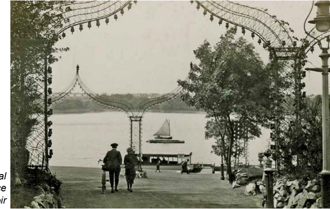
The original Victorian entrance to the reservoir
