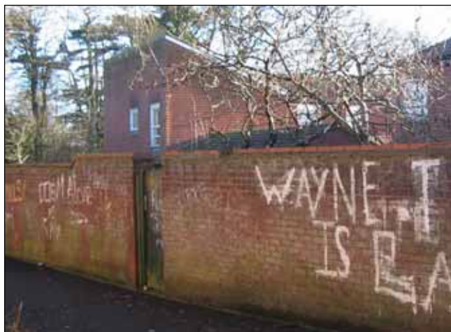
Degraded and vandalised local environment
