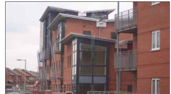
New flats being constructed at Attwood Green
