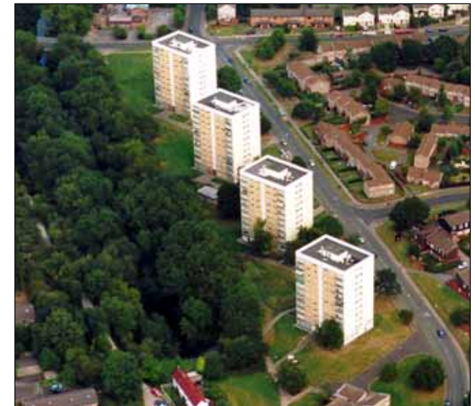
Existing blocks of flats alongside the canal
