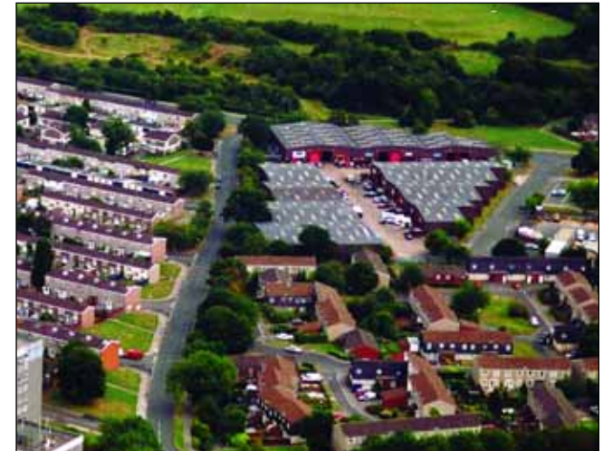
Aerial view showing Bilton Industrial Estate
