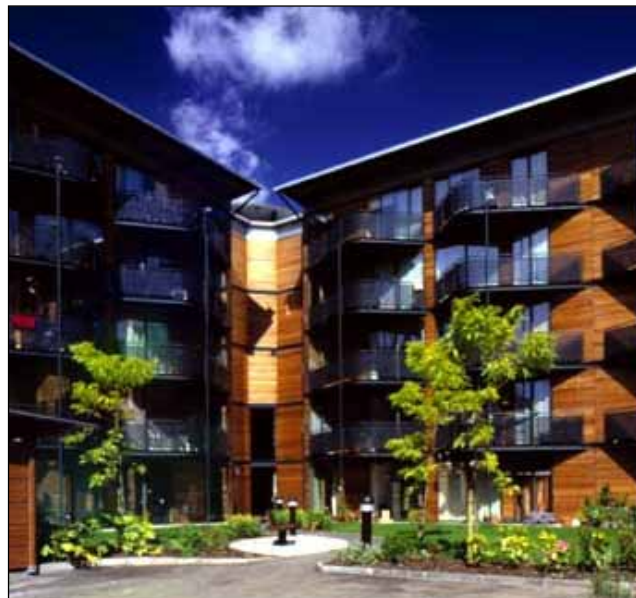
Flats constructed using prefabricated building elements
