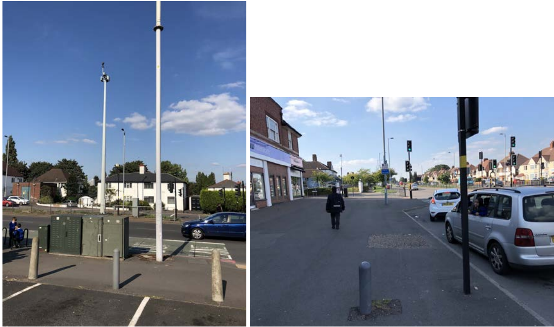
Tower Hill frontage – hard boundary treatment and telecoms units.
