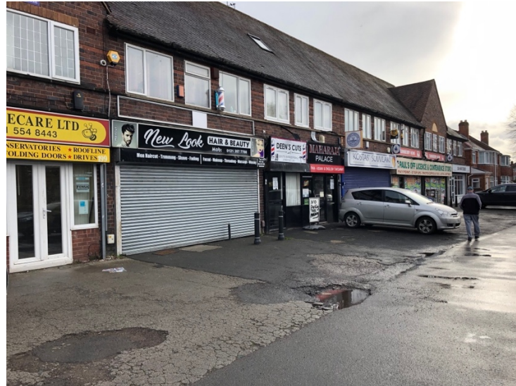
Forecourt - Turnberry Road Shops
