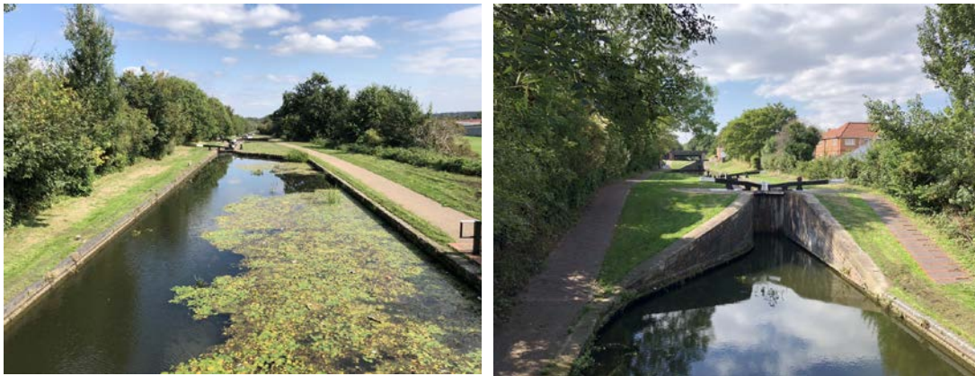
Recently improved canal and tow path adjacent to Perry Park
