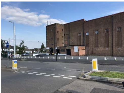
A - Unsympathetic hard landscaping and boundary treatment around the Listed Building Badshah Palace
