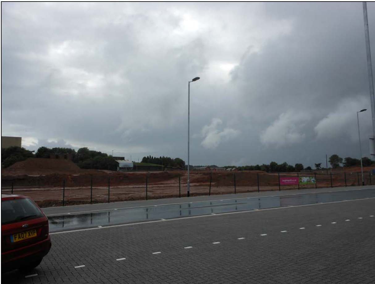
Non-Food Retail and Car Park site
