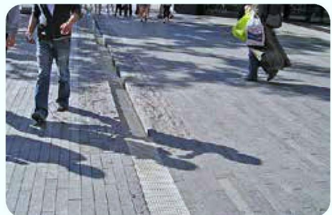
An urban rill at More London provides drainage as a multi-functional streetscape feature
