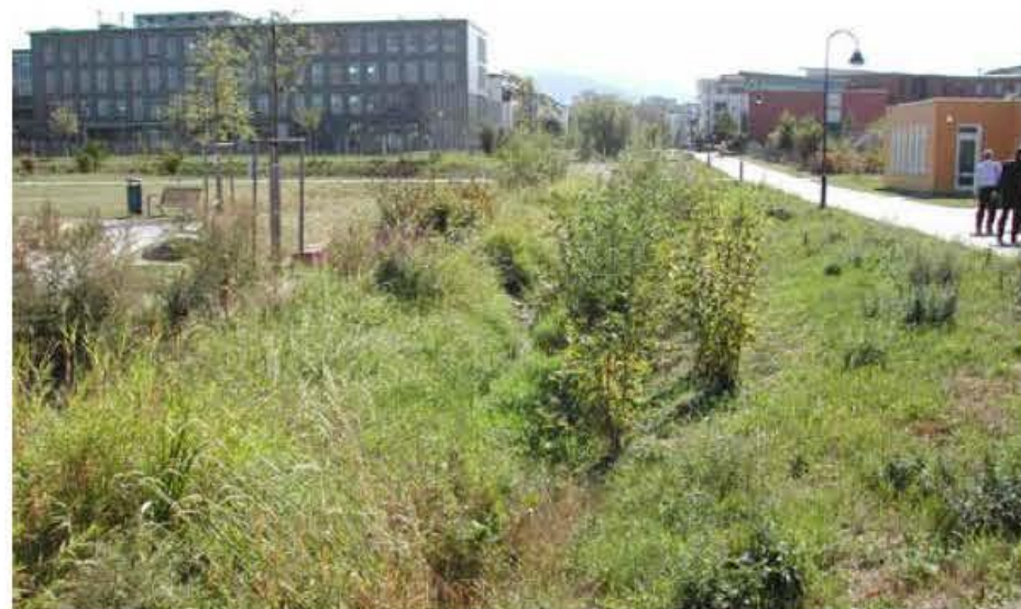
Figure 5.43 Convey swale with dense planting, Rieselfeld residential district, Freiburg, Germany
