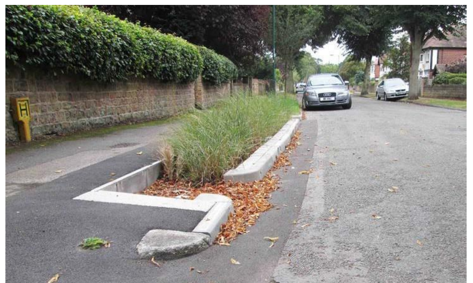
An example of ‘retrofit SuDS’ on Ribblesdale Road in Nottingham. Small strips of the kerb and pavement have been broken out and replaced with areas of planting to collect water runoff from the road.
