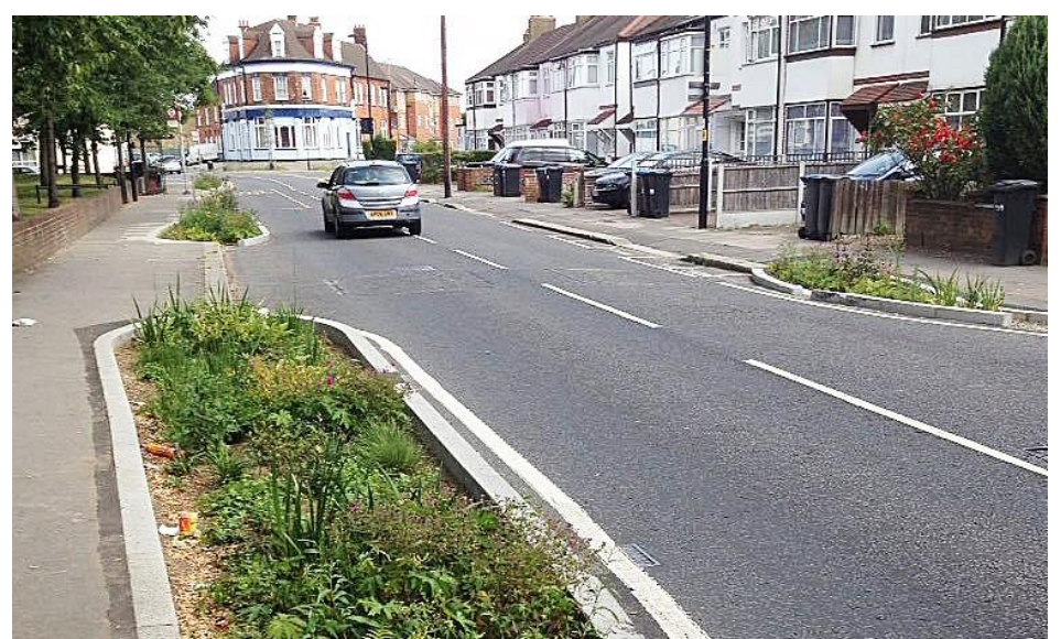
Another example of retrofitting SuDS, this time in Alma Road in Enfield. Here planted strips have been used as stormwater management, whilst also acting as traffic calming measures.
