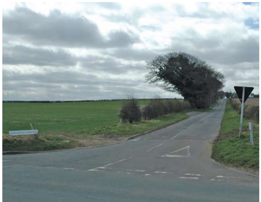
Hillwood Common Road (A2.4), constructed as part of 19th century land enclosure.
