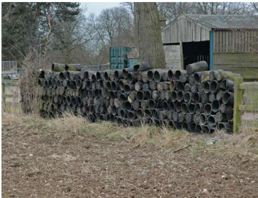
One of two stretches of walling east of Fox Hollies (C.2), constructed of crucibles used to make steel at Penns Mill.
