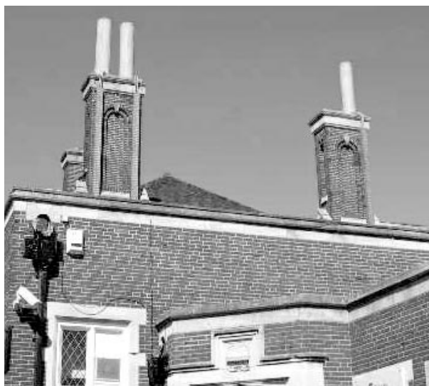
Antennae discretely designed as chimney pots
