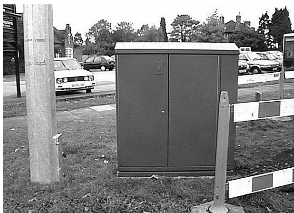
Example of a typical telecoms equipment cabinet
