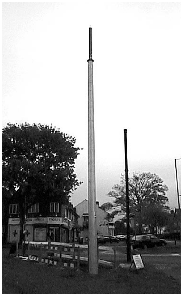
Example of a slimline mast in a mixed commercial/residential area
