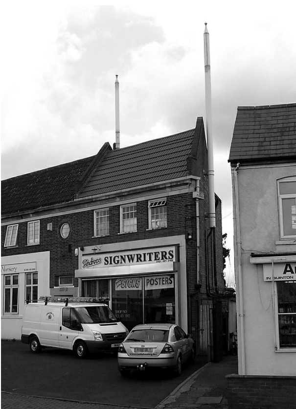
Example of antennae disguised as flagpoles
