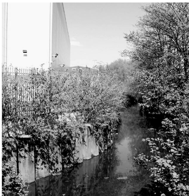
Development at the bank of the River Cole on Warwick Road.
