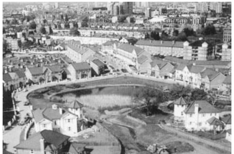
A stormwater wetland and balancing pond forms the focus of a housing redevelopment in London.
