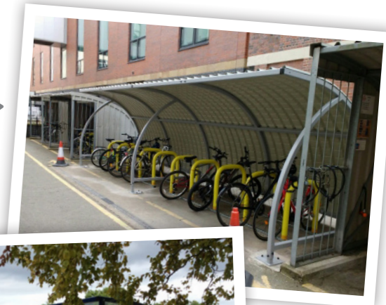
New cycle shelter at Mondelez in Bournville
