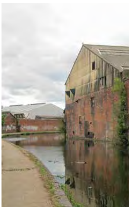
Canalside Industrial Premises
