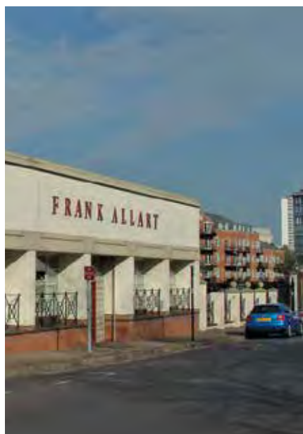
Ledsam Street Industrial Premises
