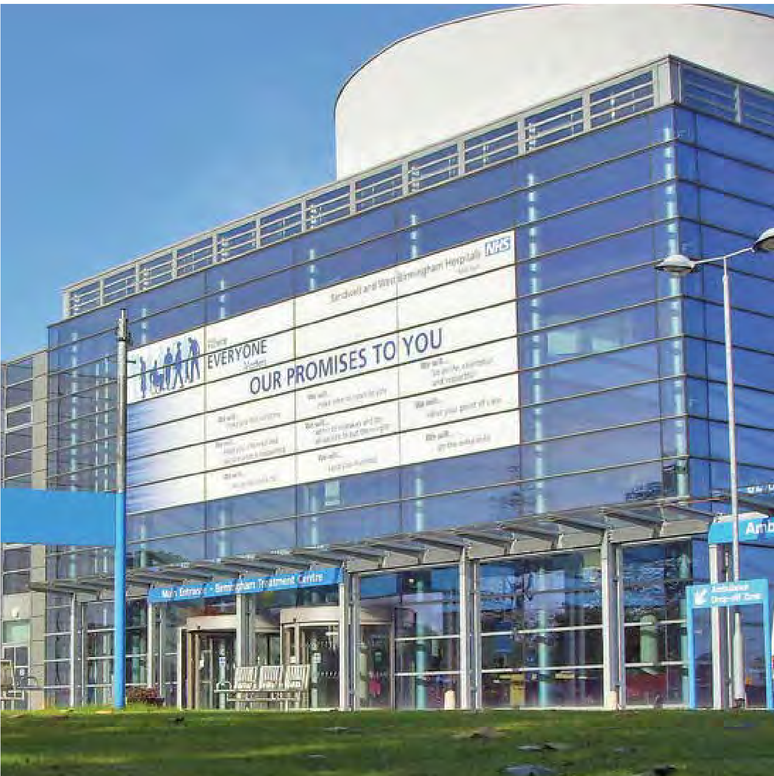
Hospital building, Dudley Road, is to be retained for health uses
