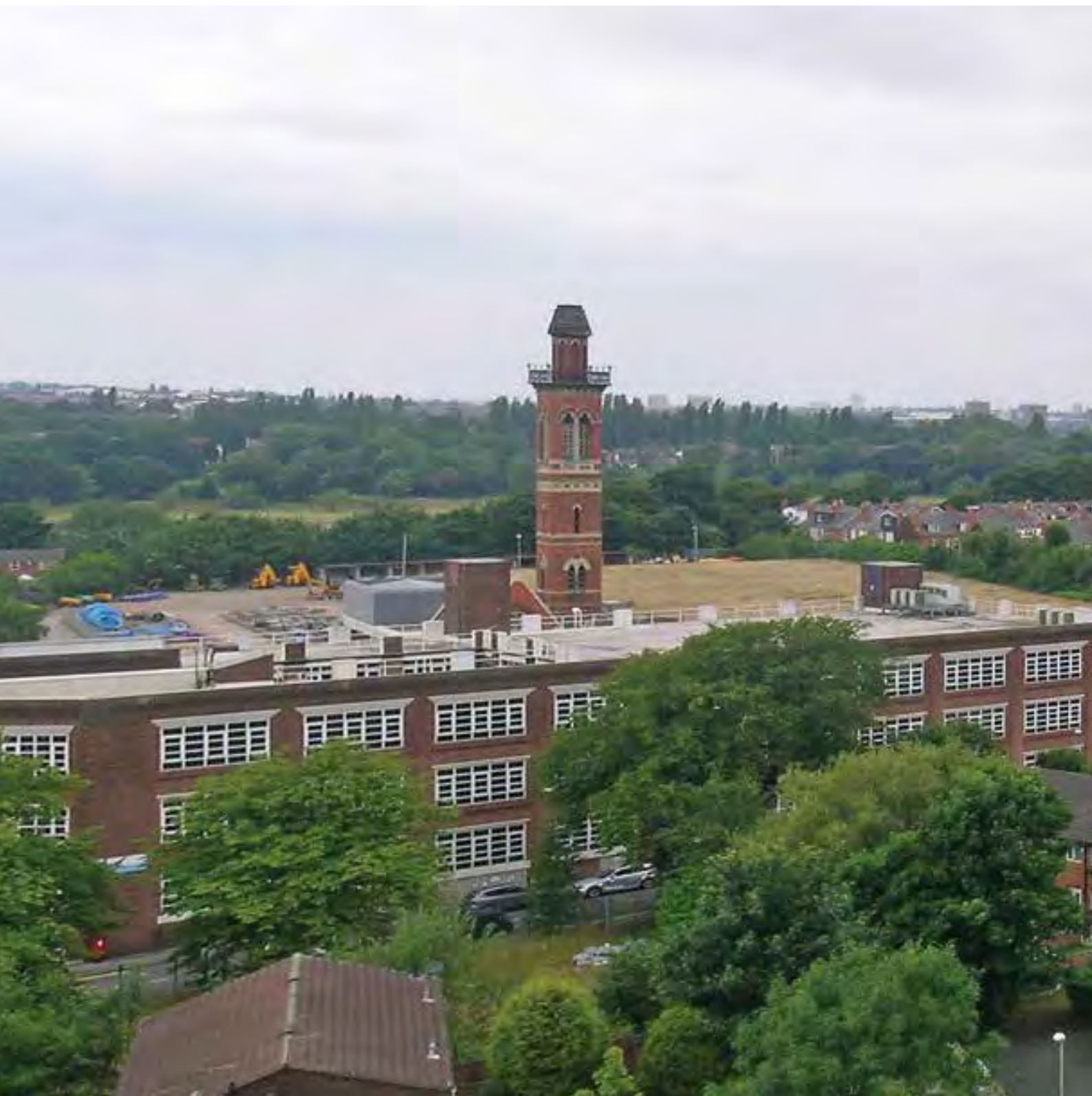
Aerial view of Waterworks Road site
