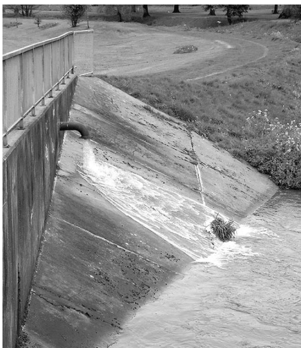
River Tame: Flood defence in Perry Hall Park.
