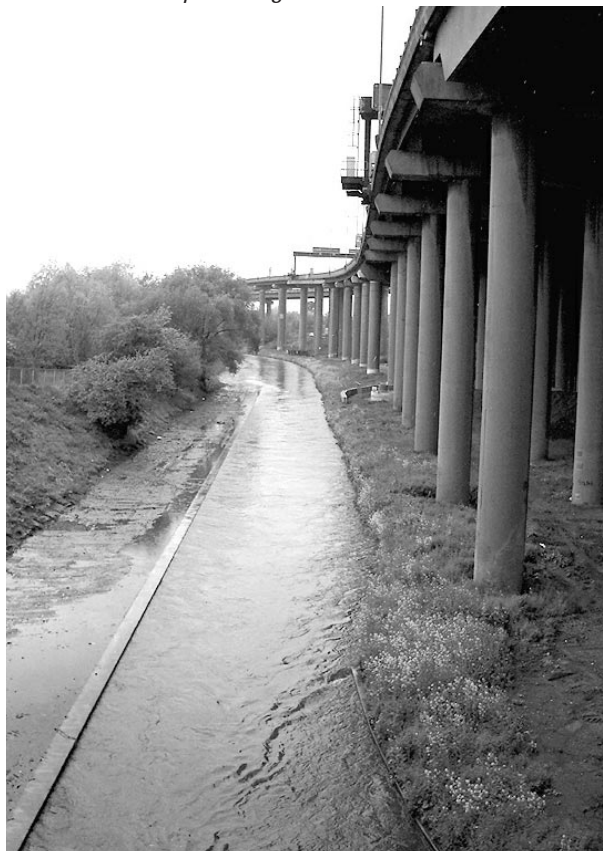
River Tame: Example of engineered channel under the M6.
