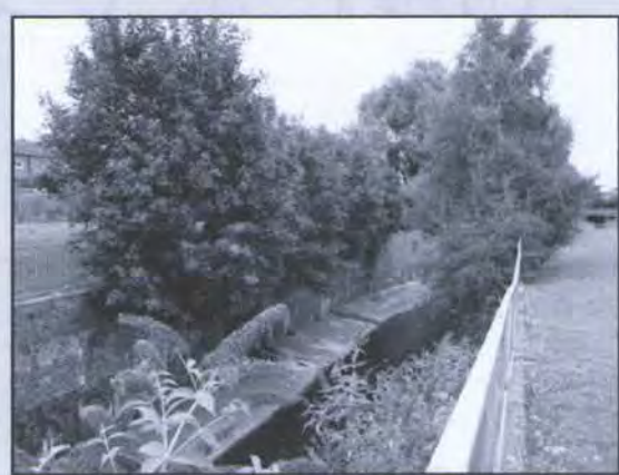
The River Rea, culverted and fenced-off, could be made into a proper river again, an asset which could be enjoyed by local people.
