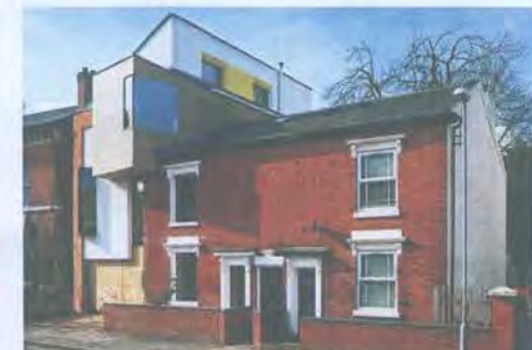
The Zero Carbon House in Tindal Street, which produces 147% of its own electrical energy needs.
