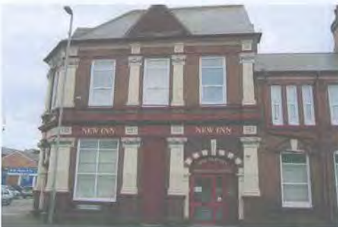
The New Inn Business Centre on Moseley Road, converted from a pub.
