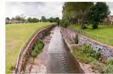
The river near Clevedon Road
