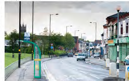
A general view of Stoney Lane, with Sparkgreen Park on the left.
