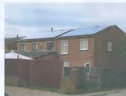
Photo-voltaic panels added to the roofs of houses on Clifton Road.
