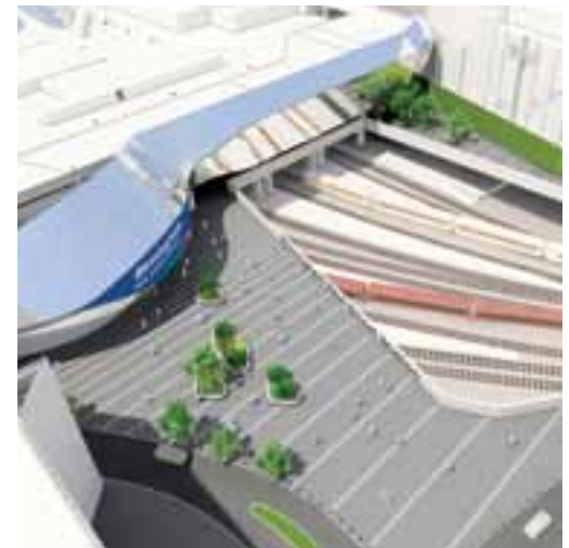
New Street Station eastern square
