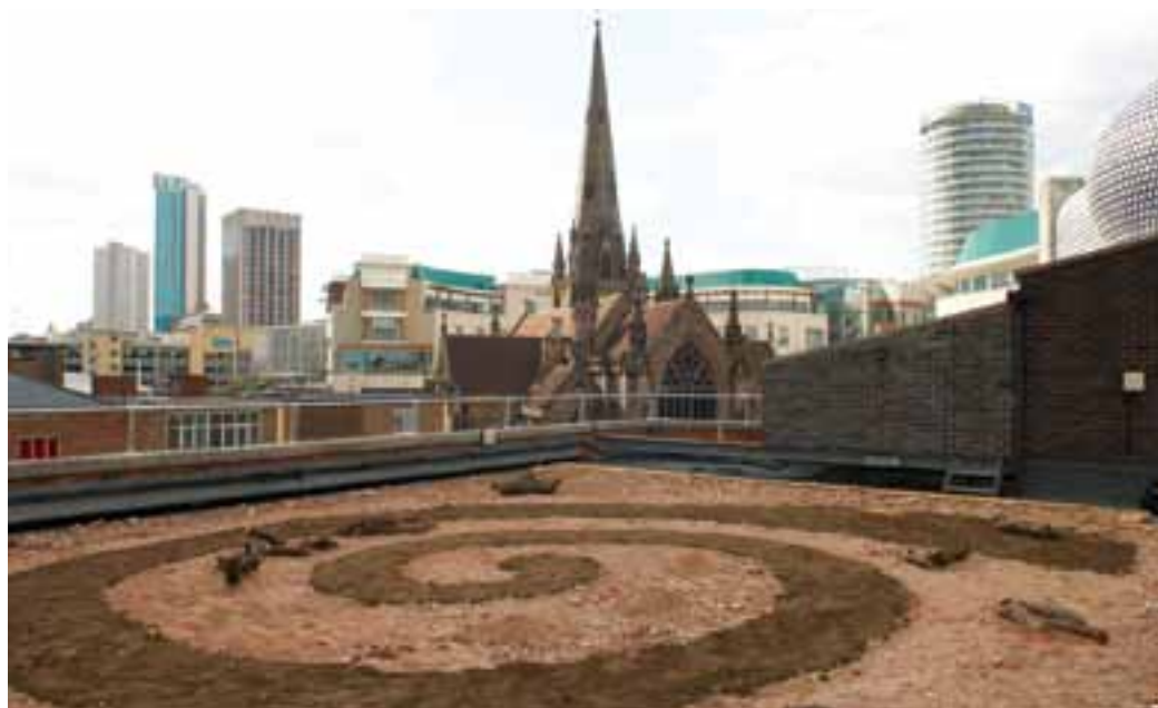
Brown roof on BSC building in Digbeth
